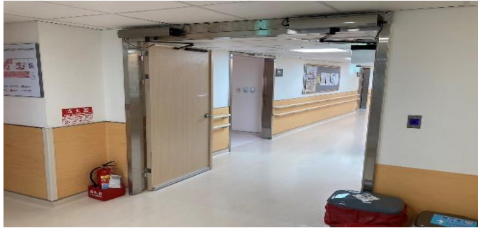
Automatic bidirectional fire door, don't need a key
